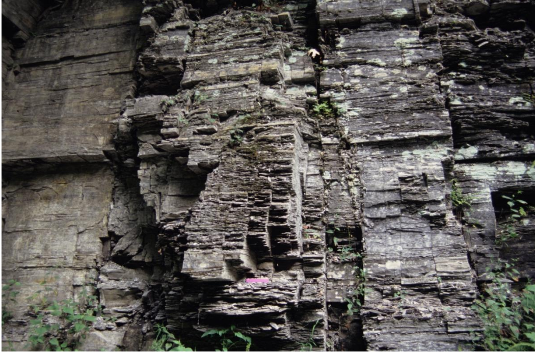
Figure 13j. Fracture intensification domain of NNW-striking fractures in the Genesee Group in Fillmore Glen (about 5 km south of the central study area. Engelder and Lash (2008) have suggested that fracture intensifications such as these mark gas chimneys. Photo by Jacobi.
