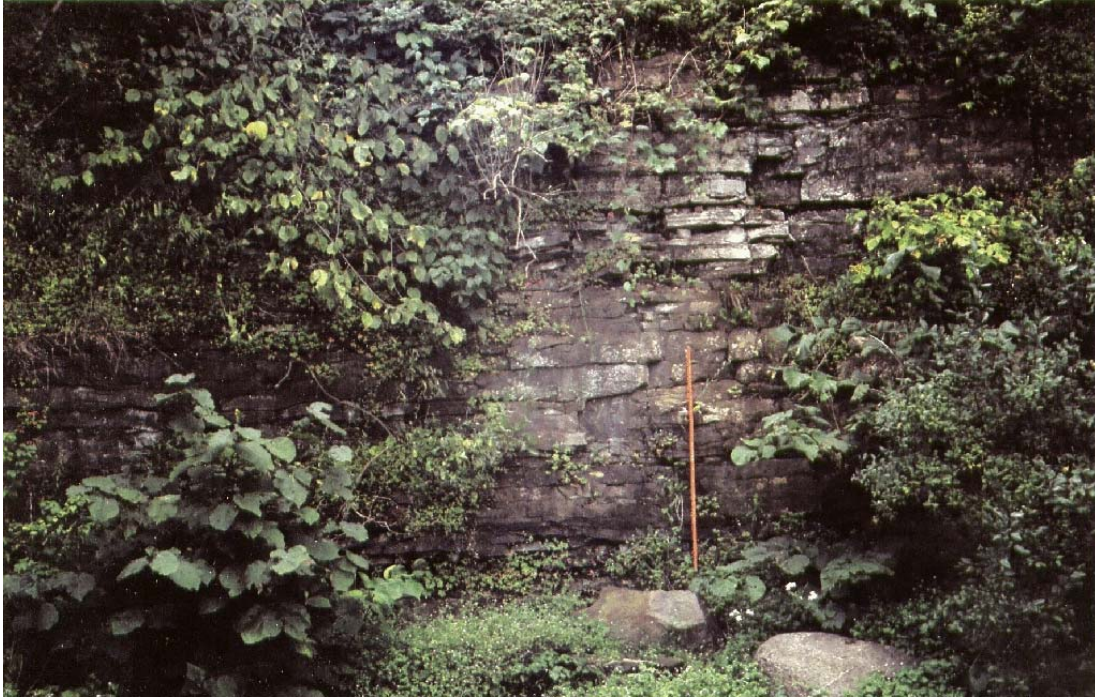
Figure 3-6 Cross Section of the Oxford Dolostone at Station OW-5. Measuring Stick 1.5 m High.
