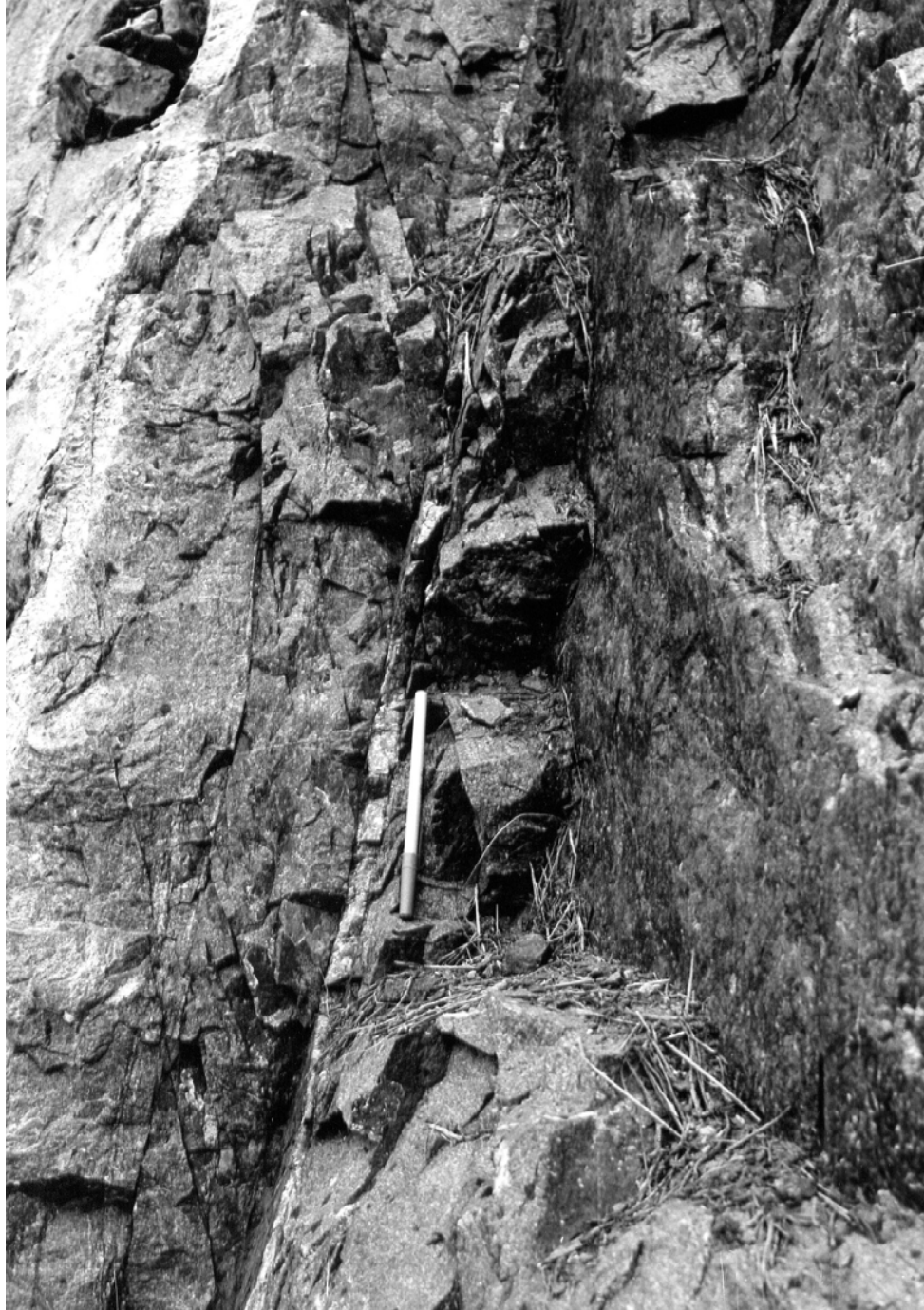
Figure 4-14 View, Looking SSW, of Normal Fault (Inclined to the Left) and Second Order Shears (Left of and Above the Pen, and Inclined to the Right) in Granite at Station E-6. Both the Fault and the Second Order Shears Parallel the Structures Seen in Figure 4-13.
